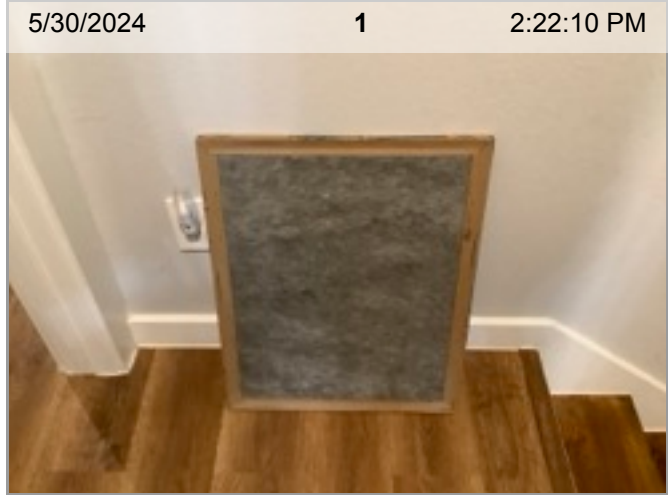
20 x 25 x 1 Air Filter Removed | Back
