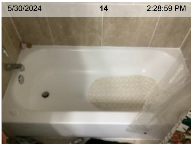
Tub/Fixture | Base of Tub
