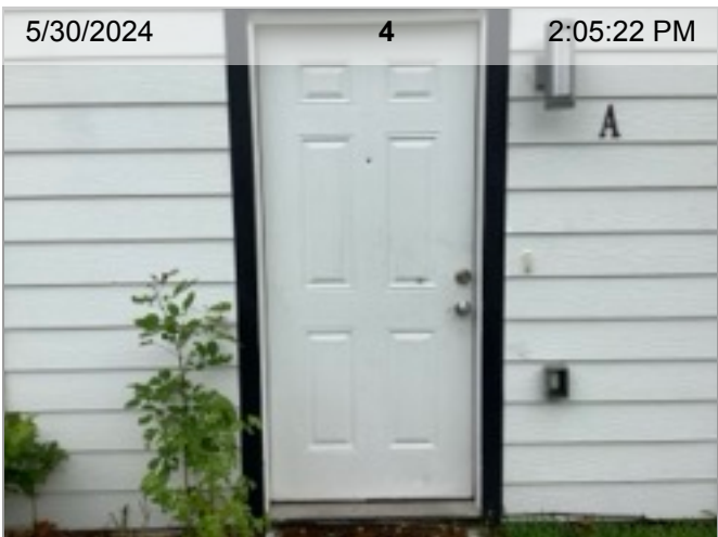
Front Door Exterior
