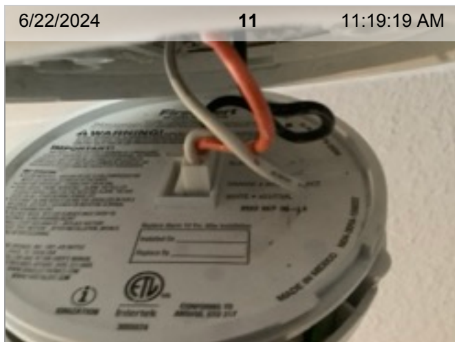
Wired Smoke Alarm (mfd 9/2022) | Smoke test: Passed | Close-up of printed manufacture date | 1.8 years old
