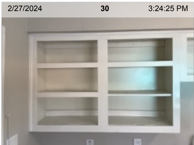
Upper Cabinets - Interior
