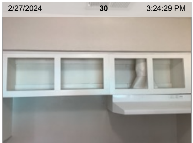
Upper Cabinets - Interior
