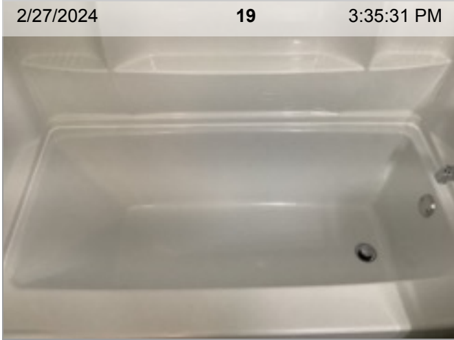
Tub/Fixture | Base of Tub
