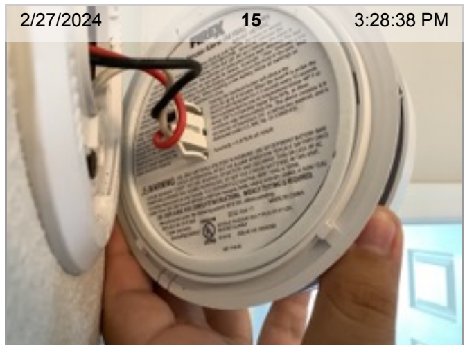
Wired Smoke Alarm (mfd 10/2022) | Smoke test: Passed | Close-up of printed manufacture date | 1.4 years old
