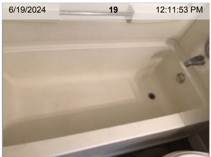
Tub/Fixture | Base of Tub
