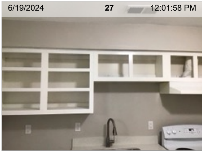
Upper Cabinets - Interior
