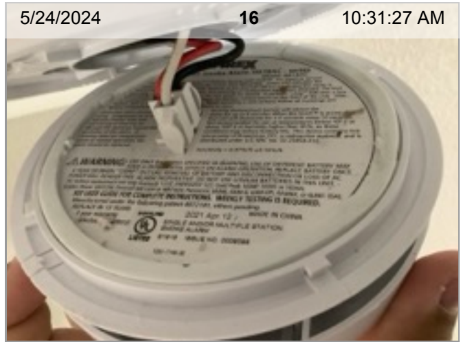
Wired Smoke Alarm (mfd 4/2021) | Smoke test: Passed | Close-up of printed manufacture date | 3.1 years old
