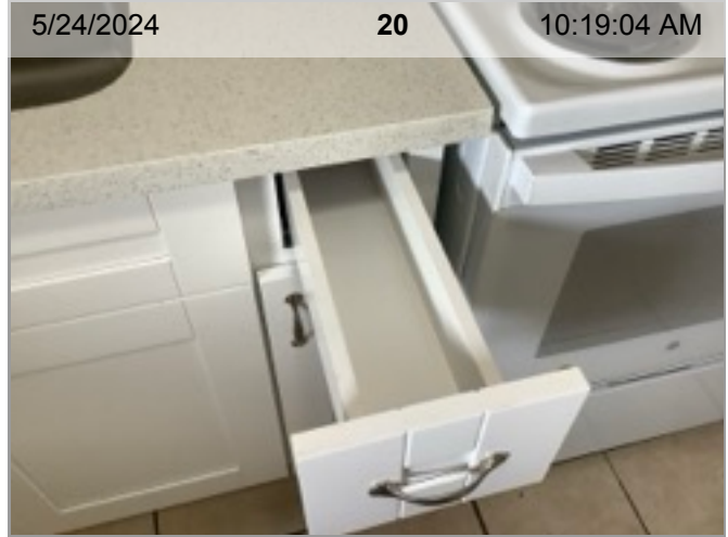
Lower Cabinets - Interior
