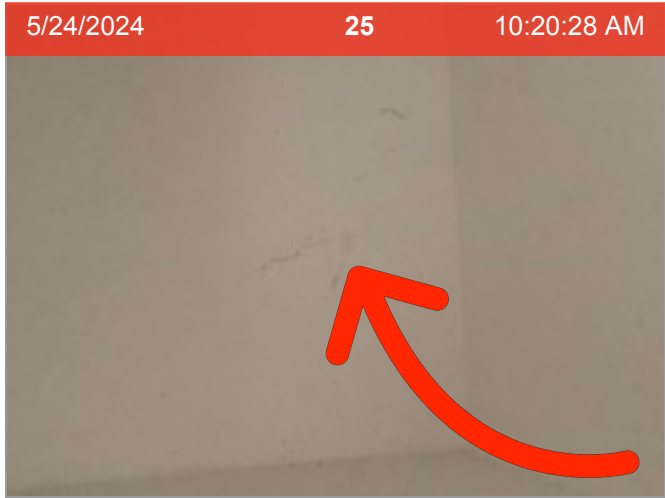
Pantry | The walls are marked up.
