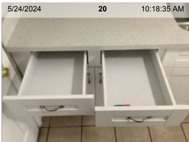
Lower Cabinets - Interior
