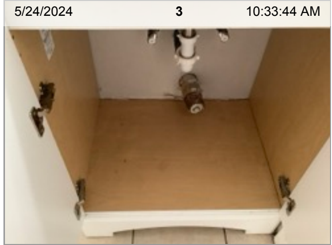
Cabinet Under Sink
