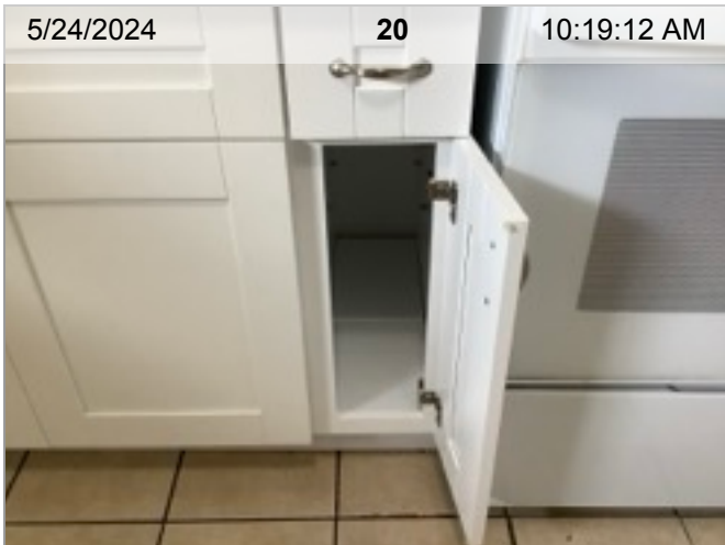
Lower Cabinets - Interior
