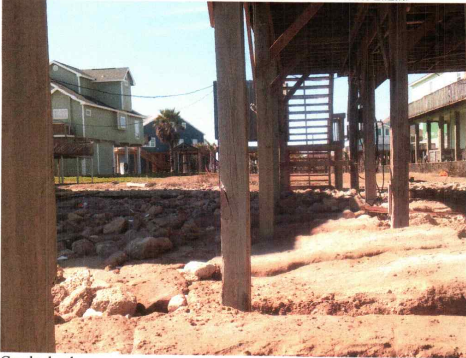
Cracked column
