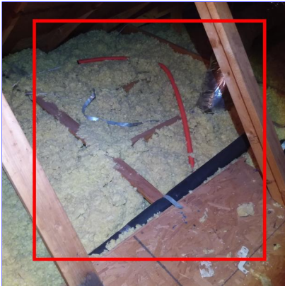
D. Item 4 (Picture) Throughout attic
