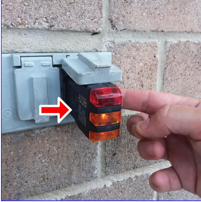
B. Item 1 (Picture) Exterior outlets
