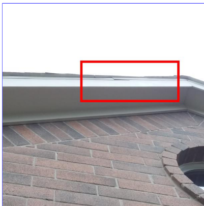
C. Item 2 (Picture) Drip edge flashing above garage
