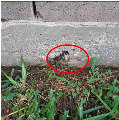
A. Item 2 (Picture) Areas around foundation perimeter
