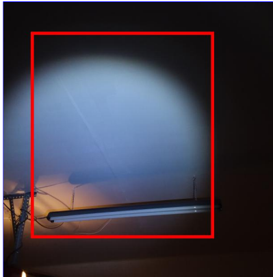
F. Item 2 (Picture) Garage
