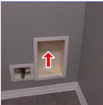
H. Item 1 (Picture) Laundry room
