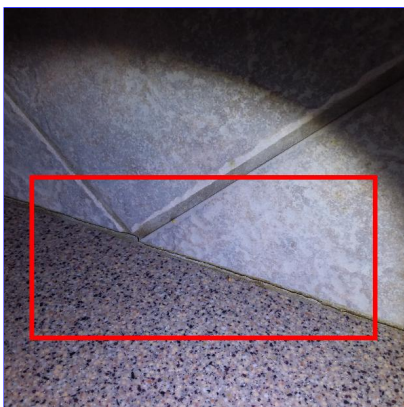
L. Item 3 (Picture) Backsplashes in kitchen in multiple areas
