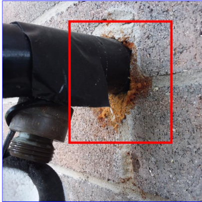
E. Item 2 (Picture) Wall penetrations
