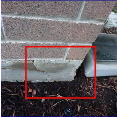
A. Item 1 (Picture) Foundation corners
