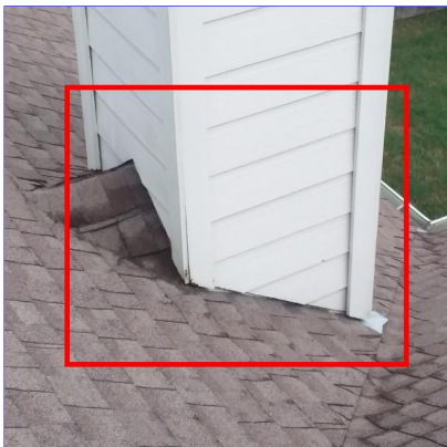
E. Item 19 (Picture) Chimney areas
