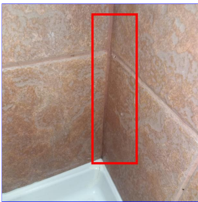
L. Item 7 (Picture) Master shower
