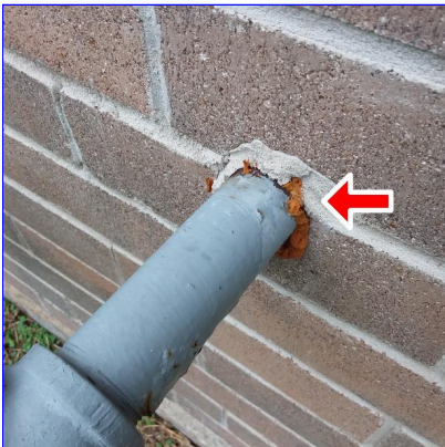
E. Item 3 (Picture) Gas meter
