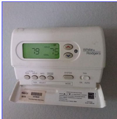
B. Item 2 (Picture) After
