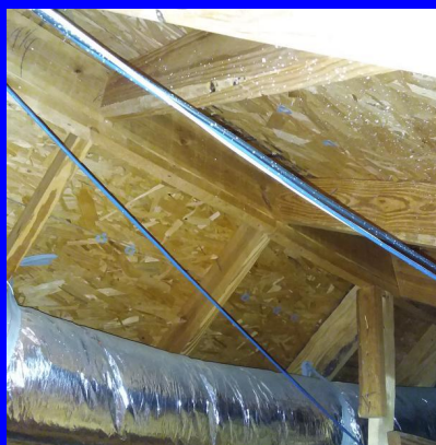
Stick built without radiant barrier
