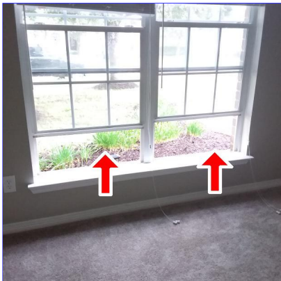
H. Item 1 (Picture) Multiple areas throughout home
