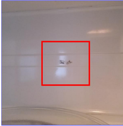
E. Item 2 (Picture) Deterioration
