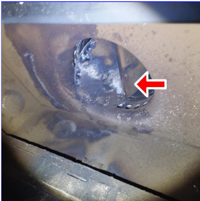
J. Item 1 (Picture) Inside fireplace
