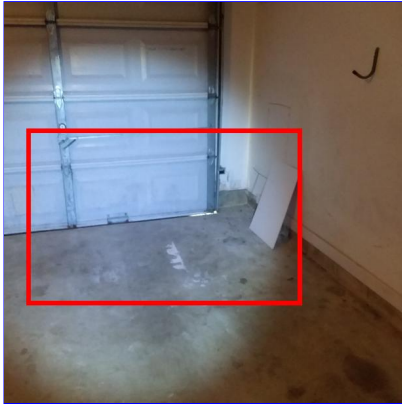
G. Item 2 (Picture) Garage door
