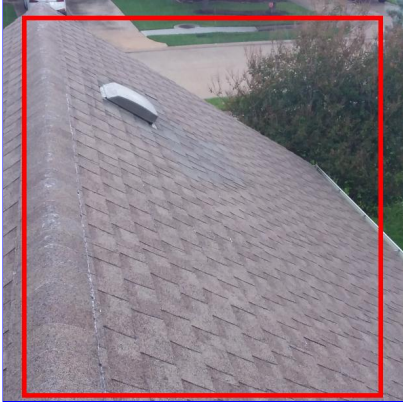
C. Item 9 (Picture) Front left
