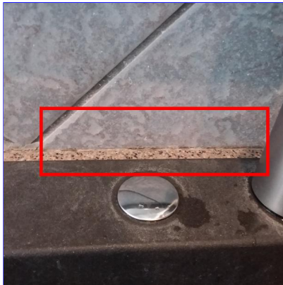
L. Item 2 (Picture) Behind kitchen sink
