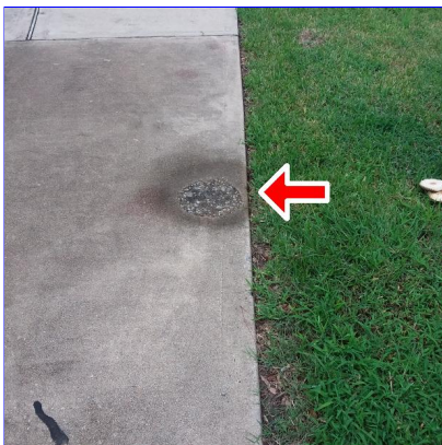
K. Item 4 (Picture) Driveway
