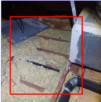
D. Item 5 (Picture) Attic
