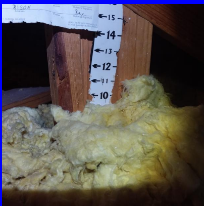
Insulation is approximately 10" deep
