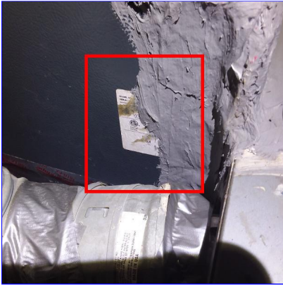
B. Item 7 (Picture) Attic unit
