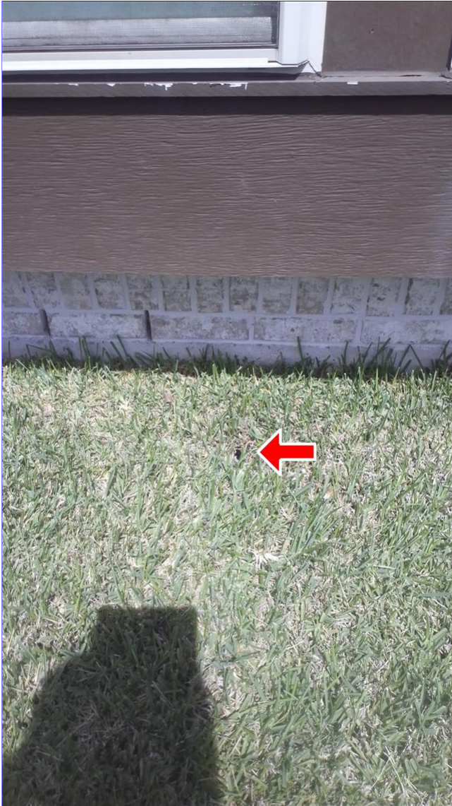
A. Item 6 (Picture) zone 4
