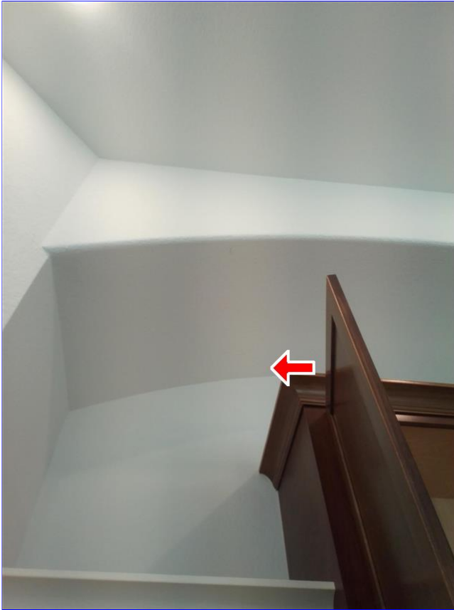
F. Item 3 (Picture) kitchen
