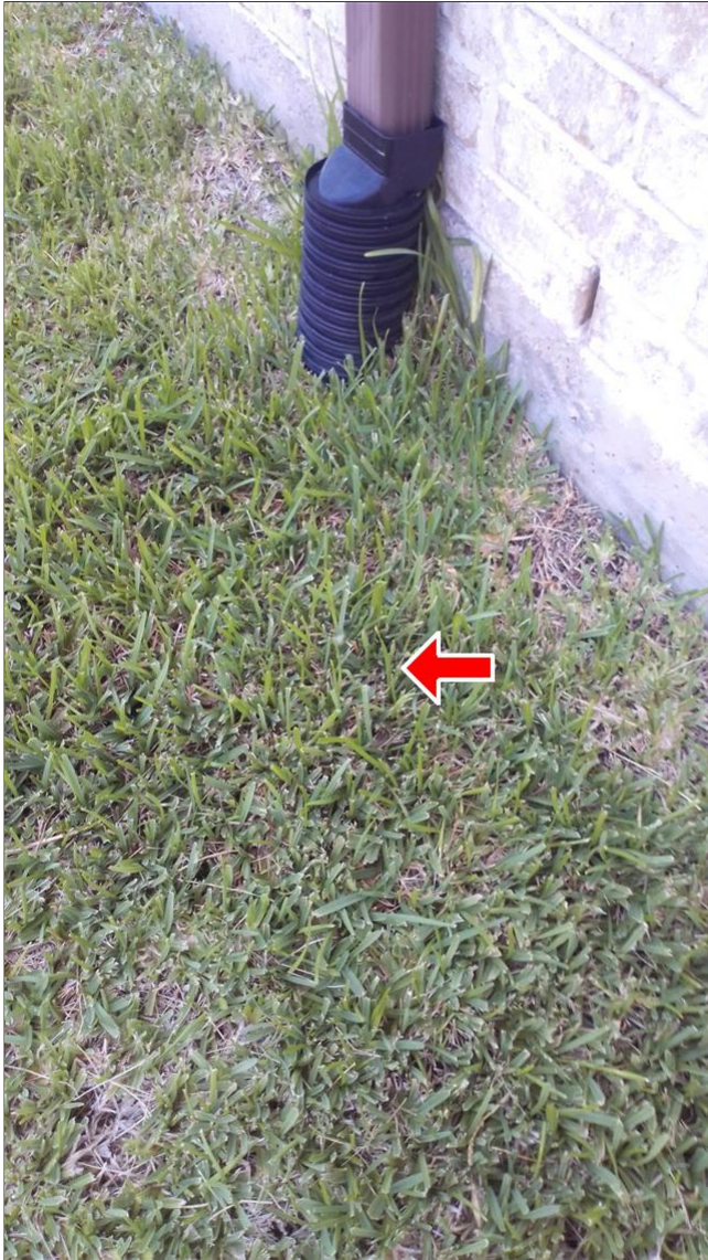
A. Item 9 (Picture) zone 5
