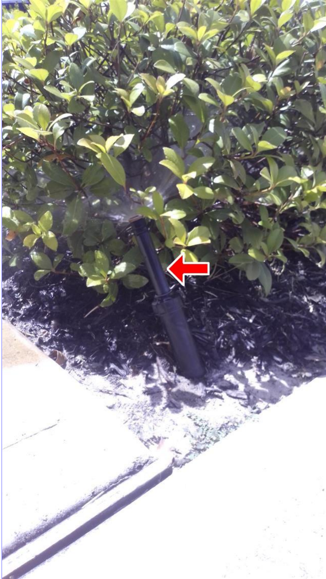
A. Item 1 (Picture) zone 1
