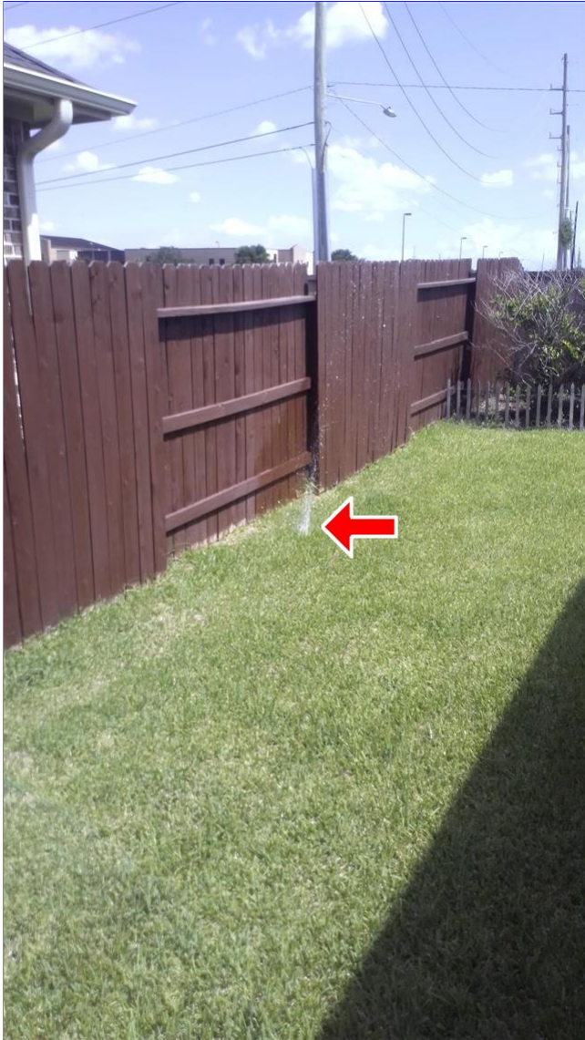
A. Item 10 (Picture) zone 5
