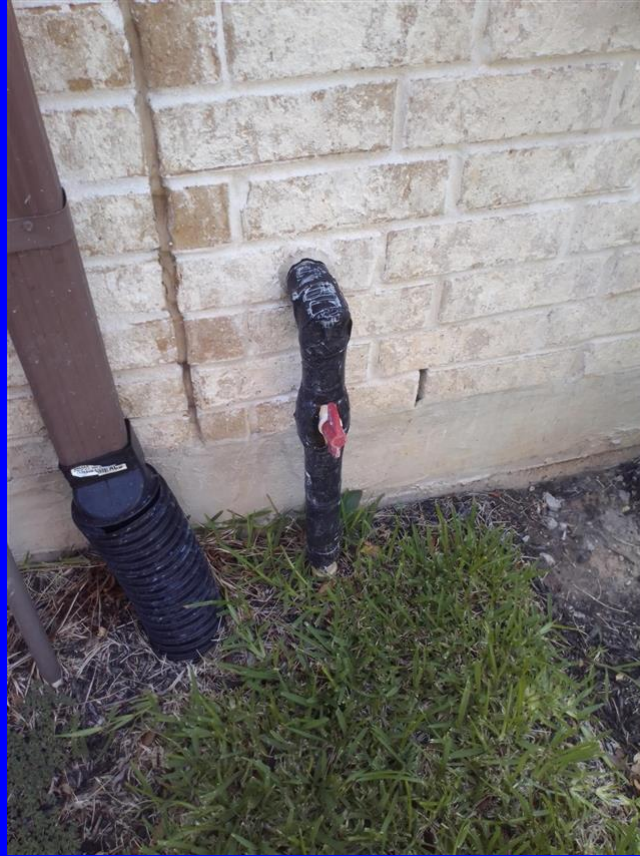
main water shut off
