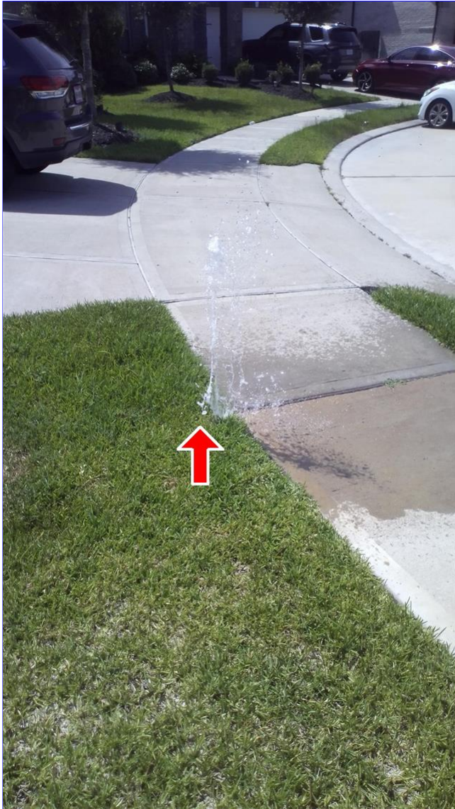
A. Item 3 (Picture) zone 2
