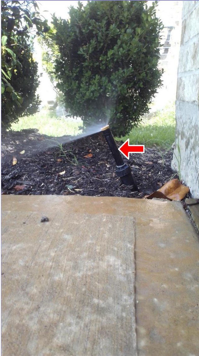
A. Item 2 (Picture) zone 3
