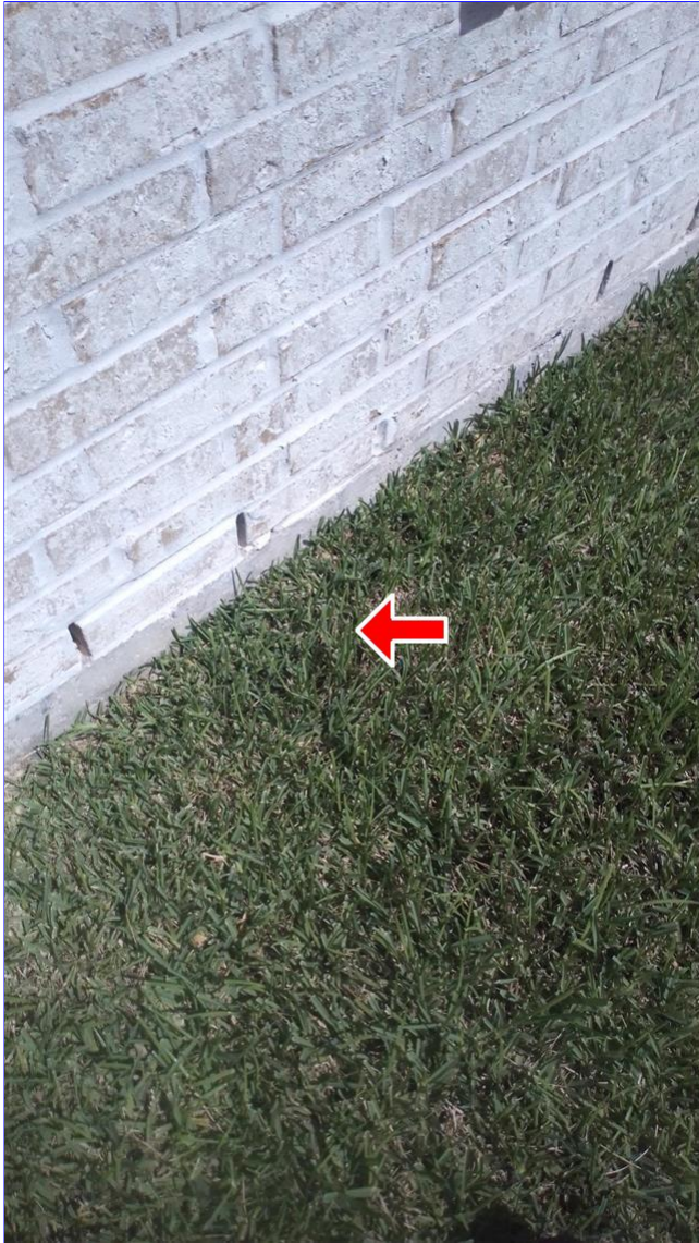
A. Item 7 (Picture) zone 4
