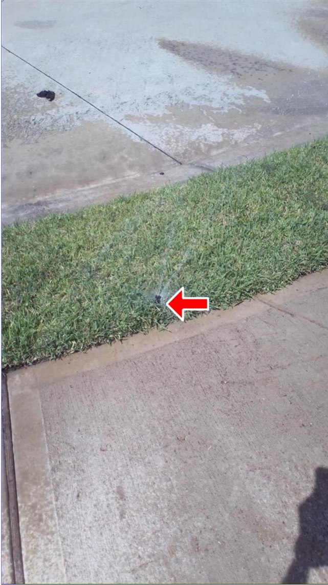
A. Item 4 (Picture) zone 2
