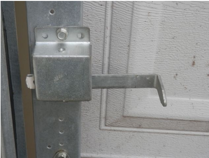
manual lock is recommended to be disabled or removed - no safety sticker at the push-button for auto-opener
