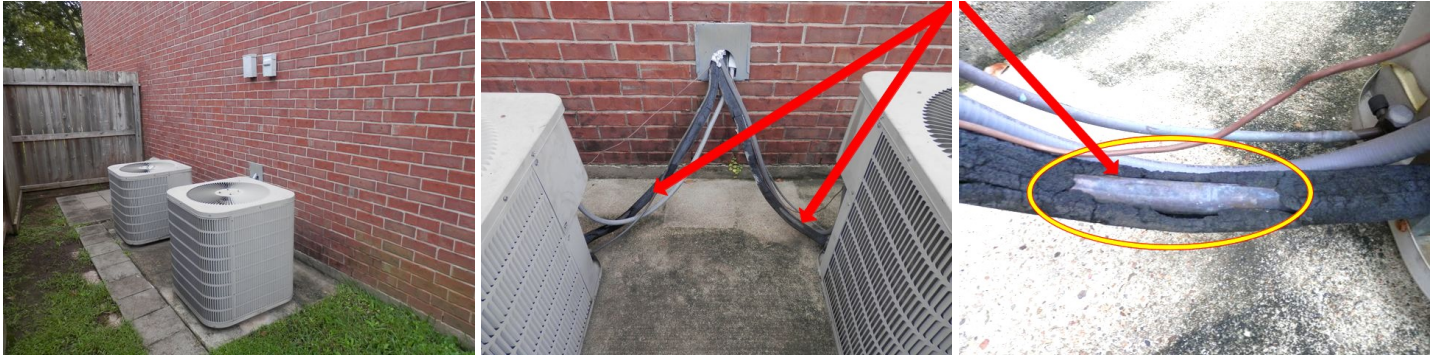
two outside a/c units with a disconnect - insulation on suction lines was damaged
