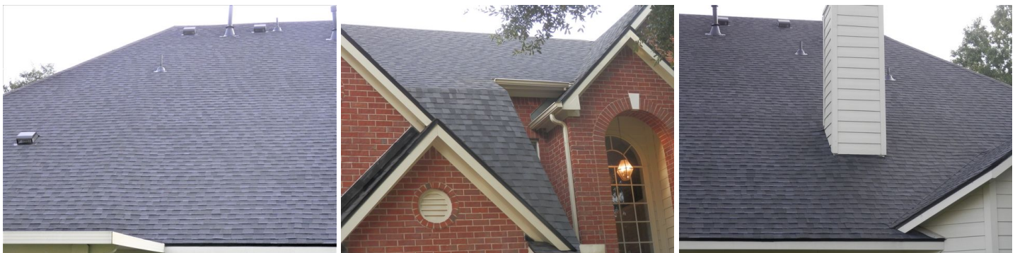
general view of the roof covering as seen from the ground
