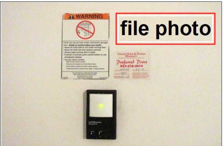
manual lock is recommended to be disabled or removed - no safety sticker at the push-button for auto-opener
