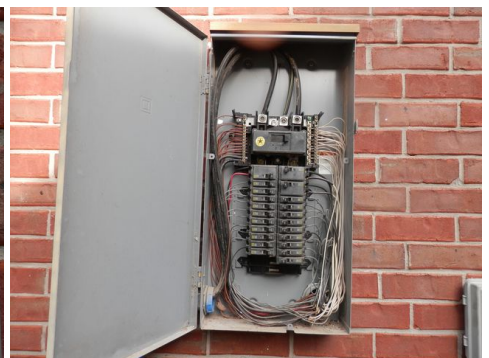
ground rod not below the soil - breakers not labeled - general view of the service panel
