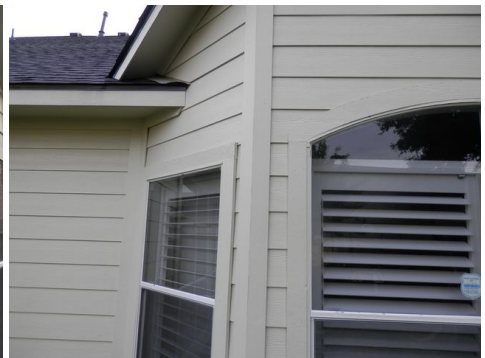
sketch of head flashing - sample of windows without head flashing
