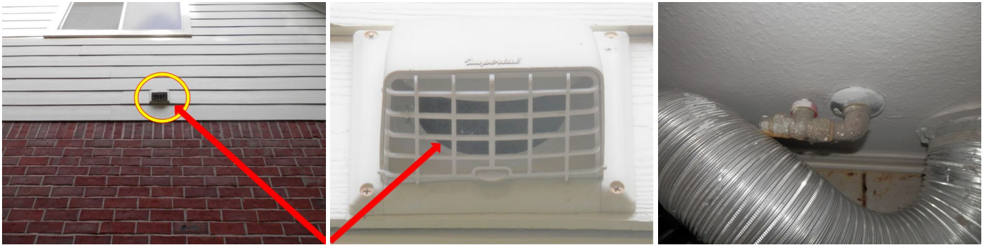
basket, snap-in cover is recommended to be moved - view of dryer vent at utility and the gas valve
