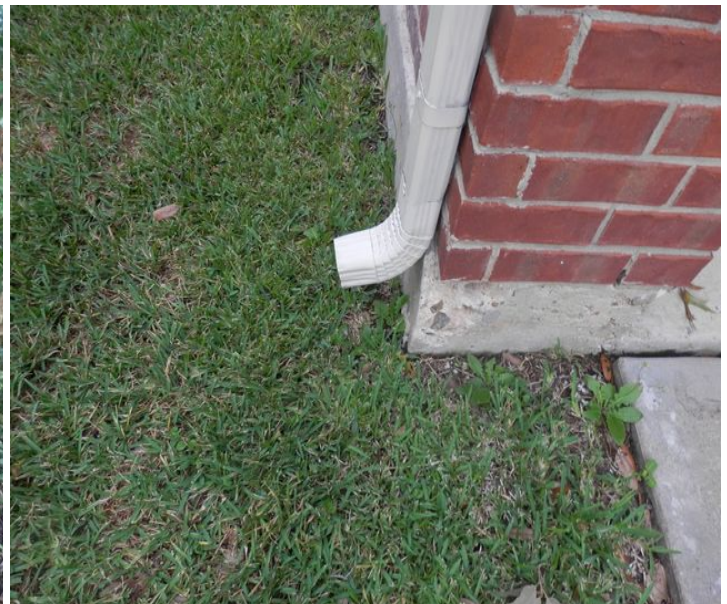
sample of high soil (at left and right of the front entry) - sample of no splash block at gutter downspout end
