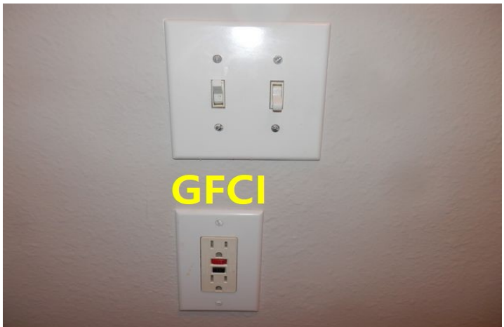
tub equipment appeared to function - GFCI was located in the toilet area of the master bath
