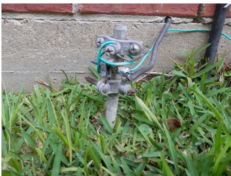
ground rod not below the soil - breakers not labeled - general view of the service panel
