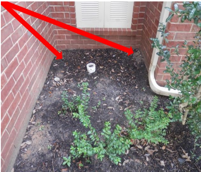
sample of high soil (at left and right of the front entry) - sample of no splash block at gutter downspout end
