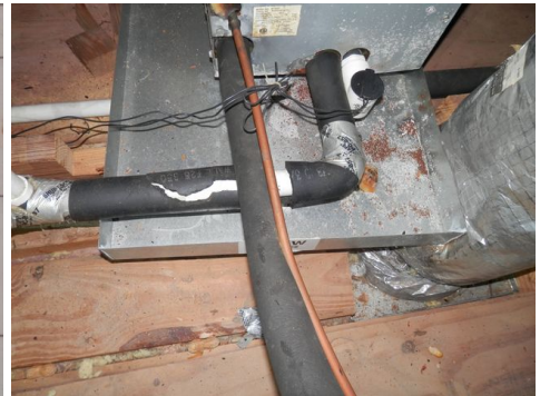
two outside a/c units with a disconnect - insulation on suction lines was damaged
