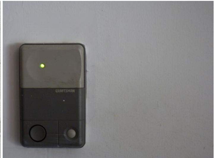
manual lock is recommended to be disabled or removed - no safety sticker at the push-button for auto-opener
