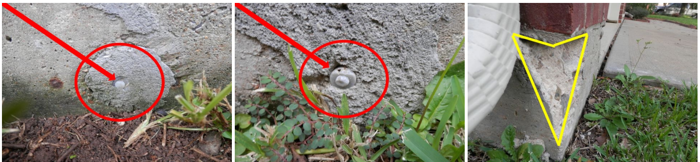
sample of exposed cable ends - sample of a wedge crack
