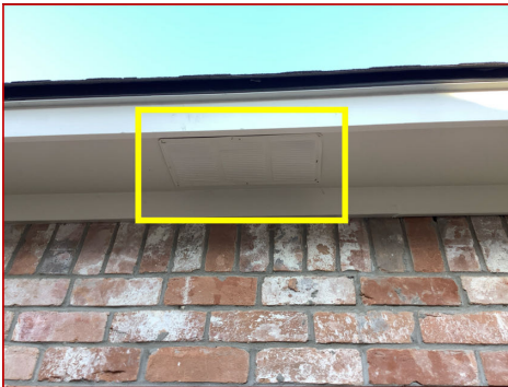
Backwards soffit vents
