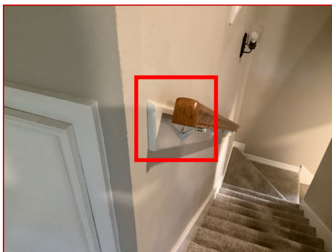
Improper termination
