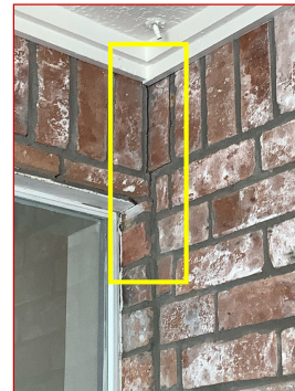
Mortar cracks
