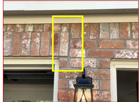
Mortar cracks
