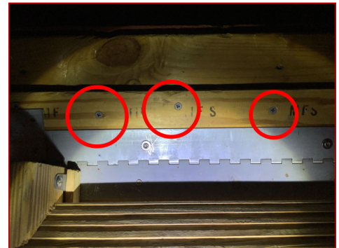
Improper fasteners
