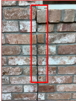
Deteriorating sealant
