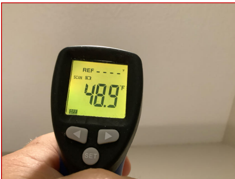
Upstairs supply temperature
