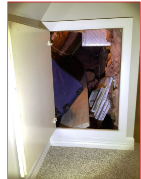
Attic access door
