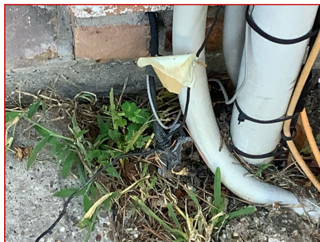
Grounding electrode and conductor
