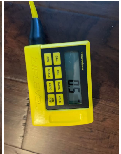
.5" higher at rear of home.
