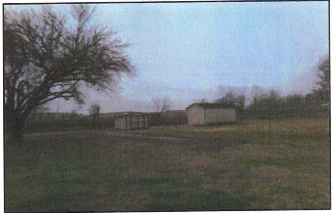
17602 Pearland Sites Rd 2 SHED & CONCRETE PAD
