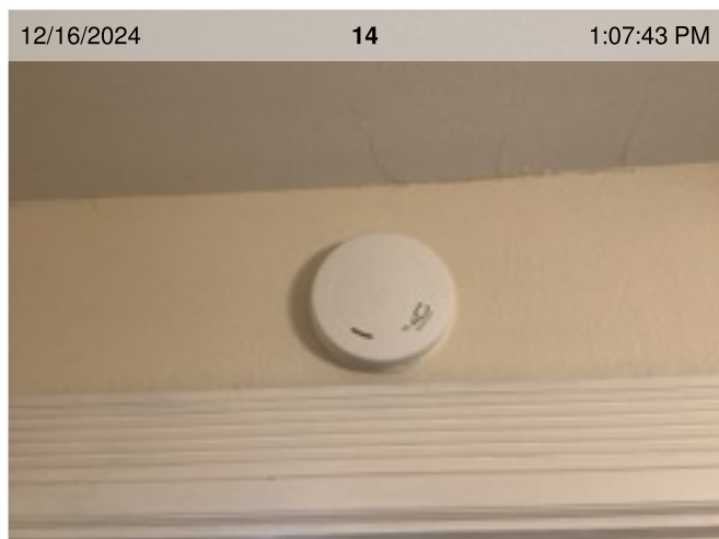
Wireless Smoke/CO Combo Smoke Alarm (mfd 2/2023) | Smoke test: Passed | Alarm in place
