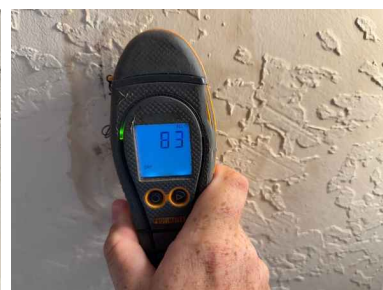
1st Floor Hall confirmed dry
