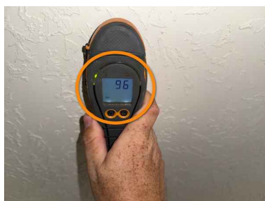
2nd Floor game room confirmed dry
