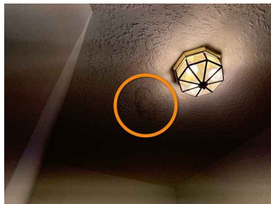
Example 1st Floor Hall
