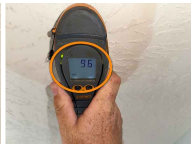
Guest Bedroom 1 confirmed dry
