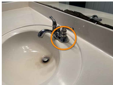
Example 2nd Floor Primary Bathroom
