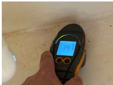
1st Floor Primary Bathroom confirmed dry
