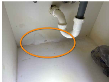
Example 1st Floor Primary Bathroom Right lavatory
