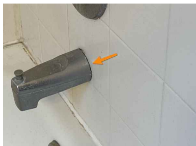
Example 2nd Floor Primary Bathroom
