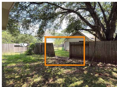
Example Rear - damage
