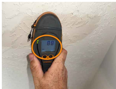
Guest Bedroom 1 confirmed dry
