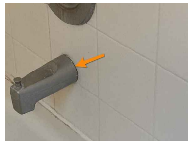
Example 2nd Floor Primary Bathroom
