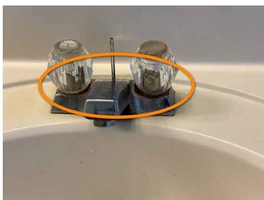
Example 1st Floor Primary Bathroom
