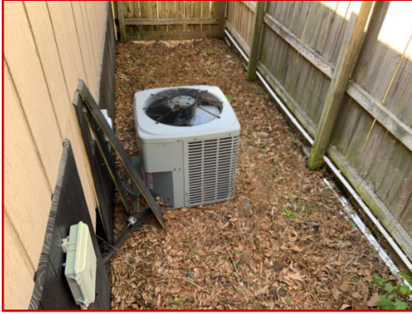
AC at rear of house
