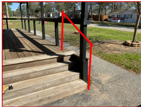
Missing handrail
