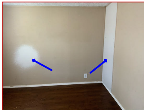
Example of wall patches
