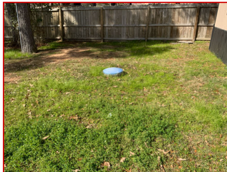
Septic not inspected
