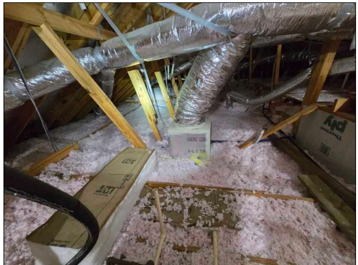
Insulation type(s): Blown fiberglass - newer style
