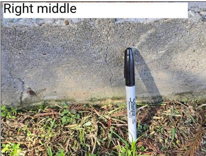
Visible crack in foundation is minor in size, but in line with left side crack. Right side.
