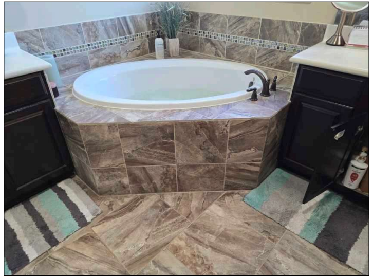
No access panel to pumps or receptacle.
