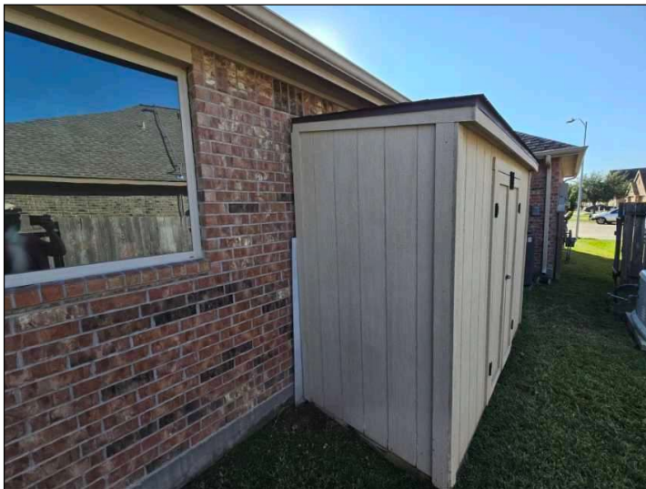
Building visually reviewed only.
