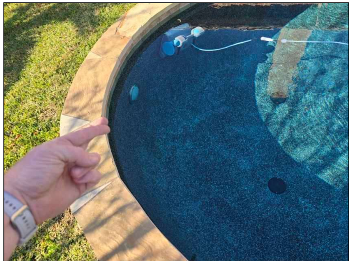
Lights did not operate. Disconnected from main panel.
