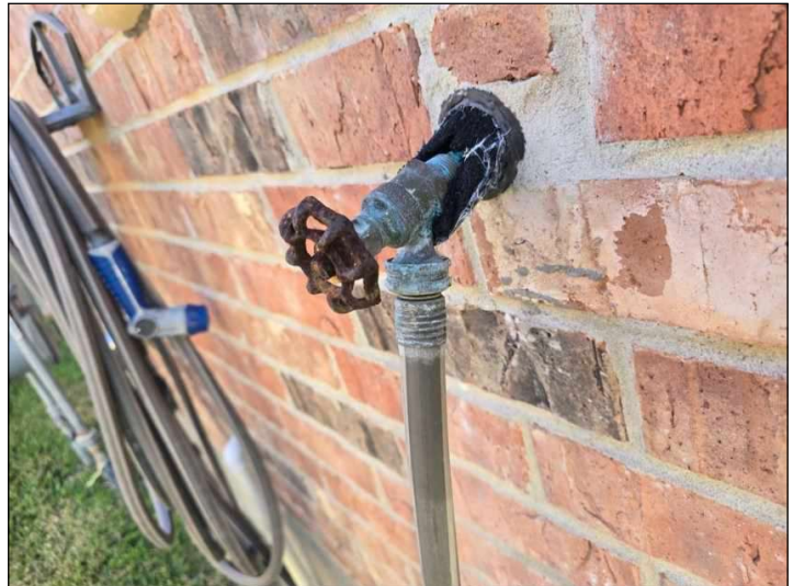
Backflow preventer not present on exterior hose bib. This will prevent contaminants from flowing back into the potable water system.
