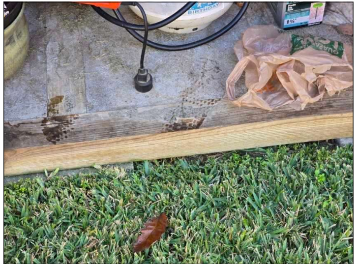
Added shed has an elevated and poured concrete base.
