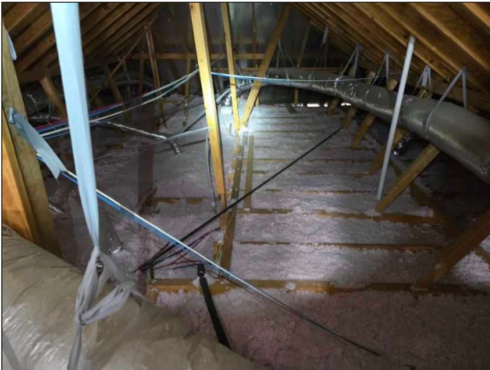
Insulation type(s): Blown fiberglass - newer style
