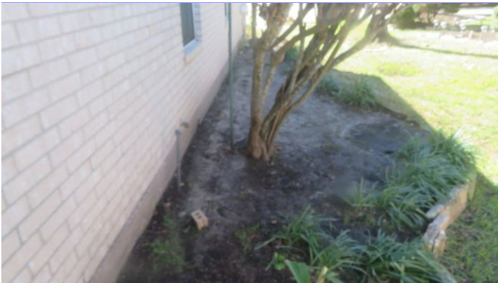
Flower beds are blocking (damming) the flow of water away from the structure. Improvements are needed.
