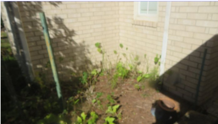
The grading should be improved to promote the flow of storm water away from the structure. This can usually be accomplished by the addition or subtraction of top soil. The ground should slope away from the structure at a rate of six inches of fall within the first ten feet. Ideally, at least 4" to 6" inches of clearance should be maintained between soil level and the top of the foundation walls. Improvements are needed.
