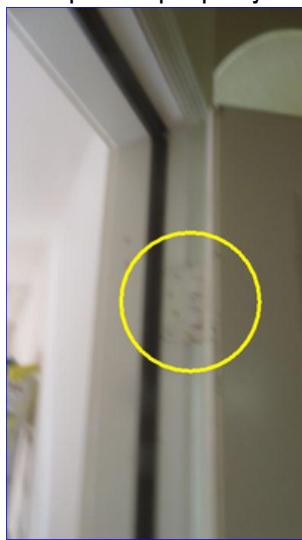
The door drags on the threshold. Adjustments to the door or threshold are recommended for the door to operate properly.
