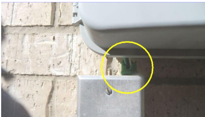
Observed damaged, missing or improper conduit. Exterior grade conduit is required for all exterior circuitry and must be sealed "Water tight" with the proper connections. Recommend repairs. (x1, sprinkler control, see pic)
