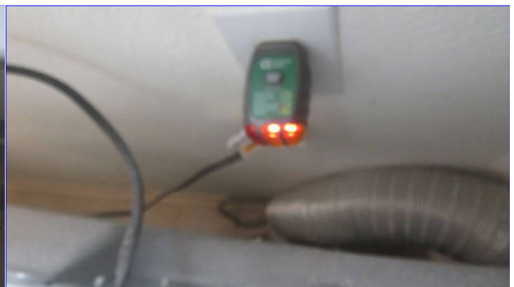
Ground fault circuit interrupter (GFCI) outlet protection was not observed at the required following outlet(s). Receptacle(s) or breakers should be replaced with proper GFCI receptacle(s)/ breakers.
