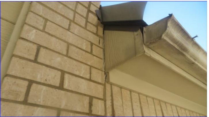
The roof gutters should be cleaned. Observed excessive debris in the gutter system. Debris can clog drains allowing water to back up, causing water intrusion of the structure. Recommend regular cleaning of all drainage systems.
