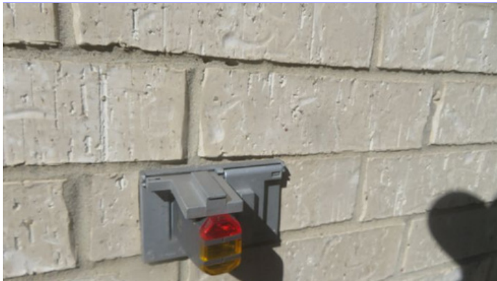
Exterior outlets are required to be weather sealed, and sealed to the surface they are mounted to. Outlets were not sealed in some areas. This is a "Shock Hazard". Repairs, can be done by installing a sealed (bubble type) outlet cover to the original outlet junction box and properly sealing it to the wall. (all)
