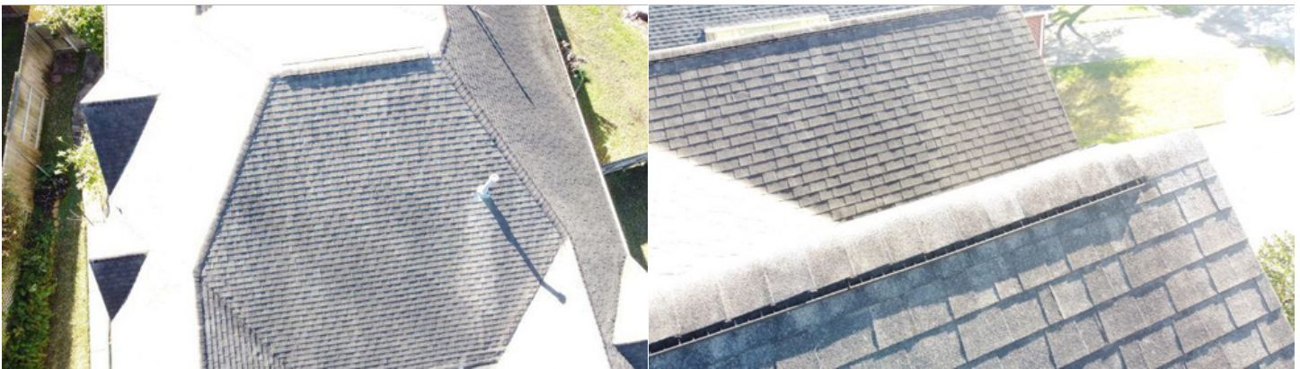
View of the Roof.
